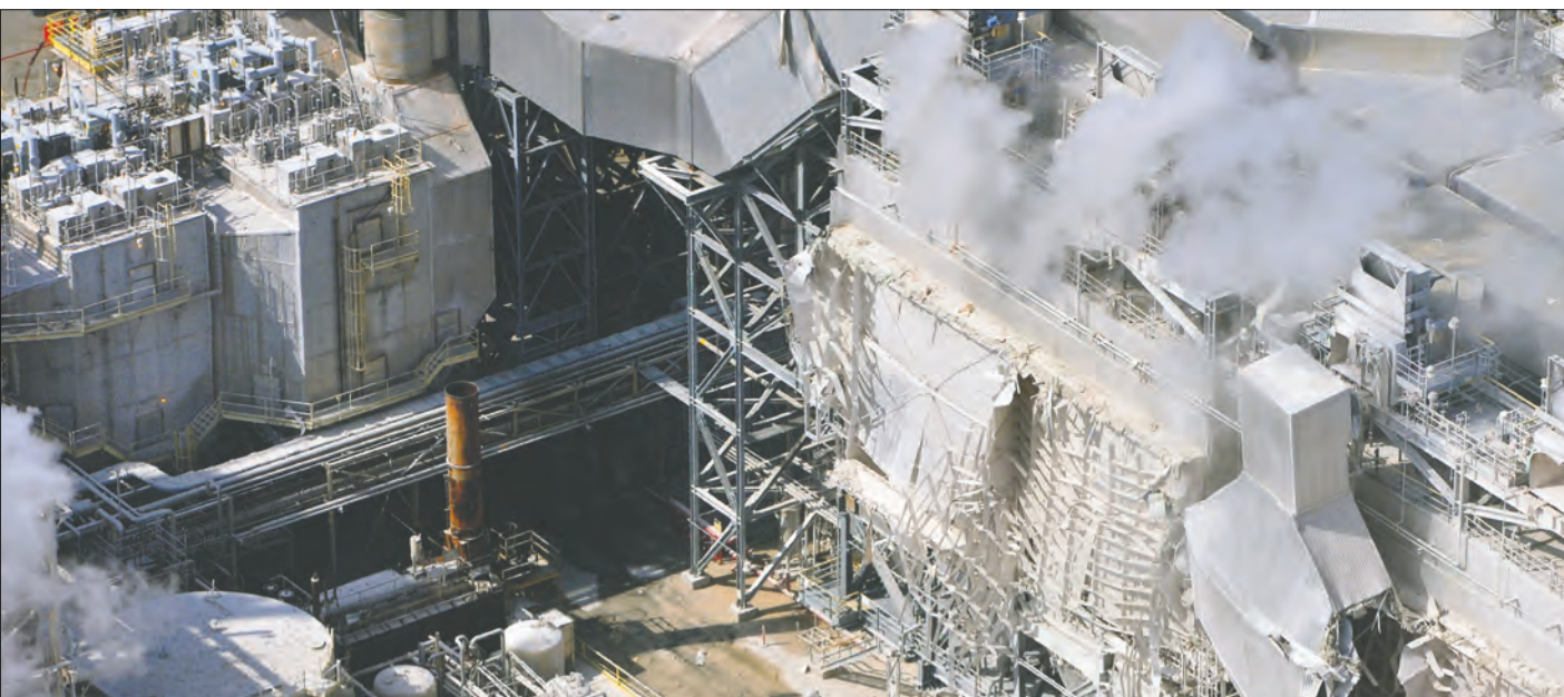
A structure is damaged after an explosion in a processing facility at the ExxonMobil refinery Wednesday in Torrance, Calif. A small ground fire was quickly extinguished and the facility's flare system was triggered for safety reasons. Two workers suffered minor injuries.
