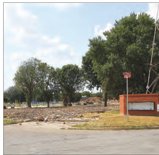
The damaged nursing home near the blast radius of the West fertilizer plant explosion has been demolished and removed. Photo taken on August 22 in West, Texas.
