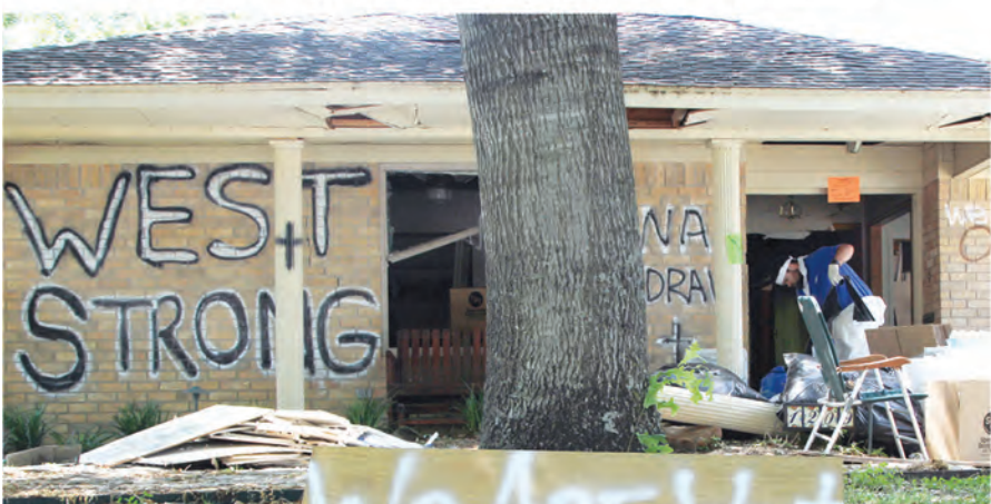
Travis Taylor | Lariat Photographer Workers clear out the inside of a damaged home in West on Monday, April 29, 2013.
